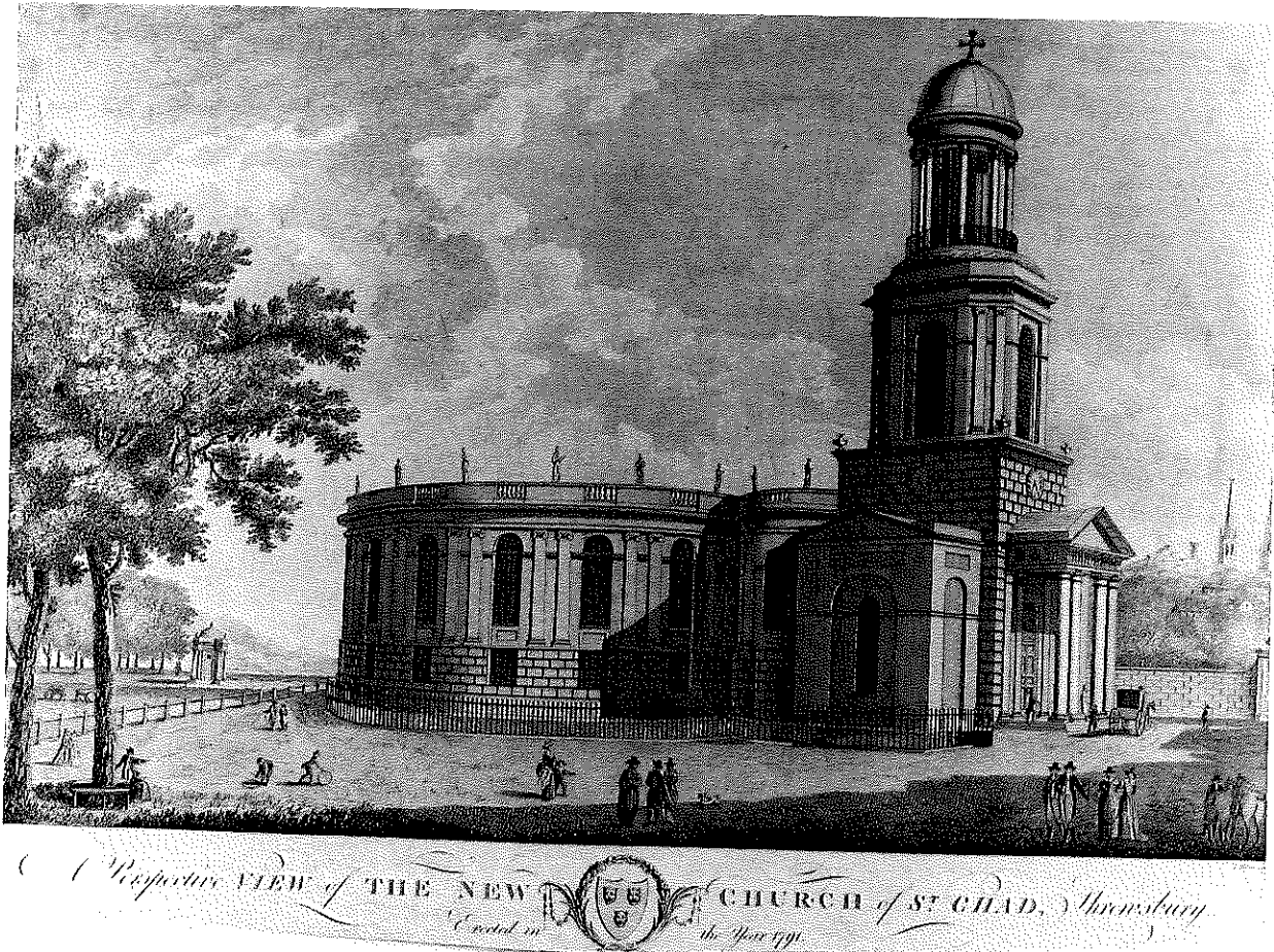
PLATE 13 ST CHAD'S, SHREWSBURY, 1789-92, DESIGNED BY GEORGE STEUART. 'A PERSPECTIVE VIEW' DRAWN BY THE ARCHITECT AND ENGRAVED BY T. MILLER, DATED 31 OCTOBER 1791 (SRR: NEG. B831).
