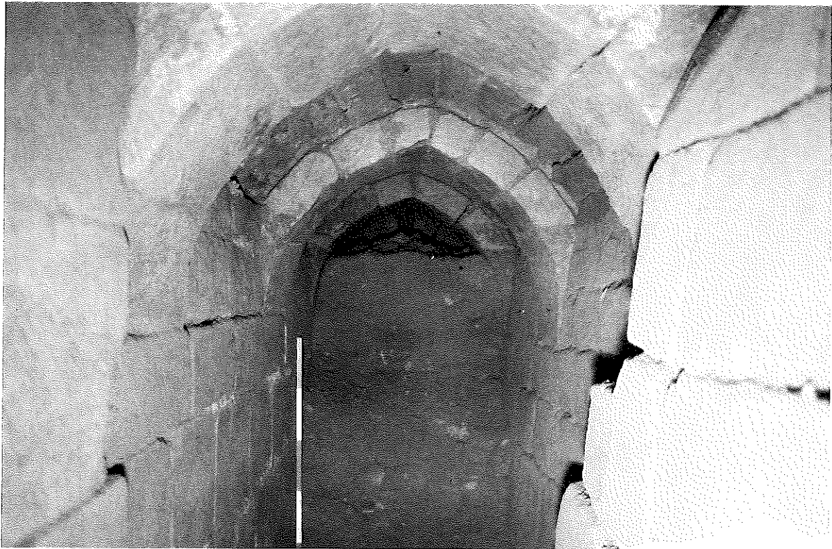
PLATE 9 STRUCTURE 3. THE CULVERT (F87). INTERIOR VIEW (J STERENBERG)
