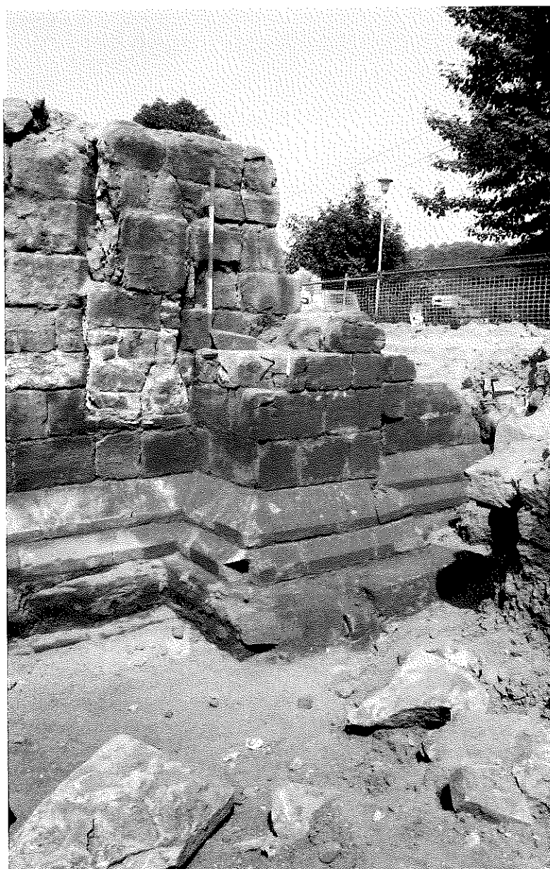
PLATE 6 STRUCTURE 1. BUTTRESS (F104) ON SOUTH SIDE OF BUILDING, VIEWED FROM THE SOUTH. (J STERENBERG)
